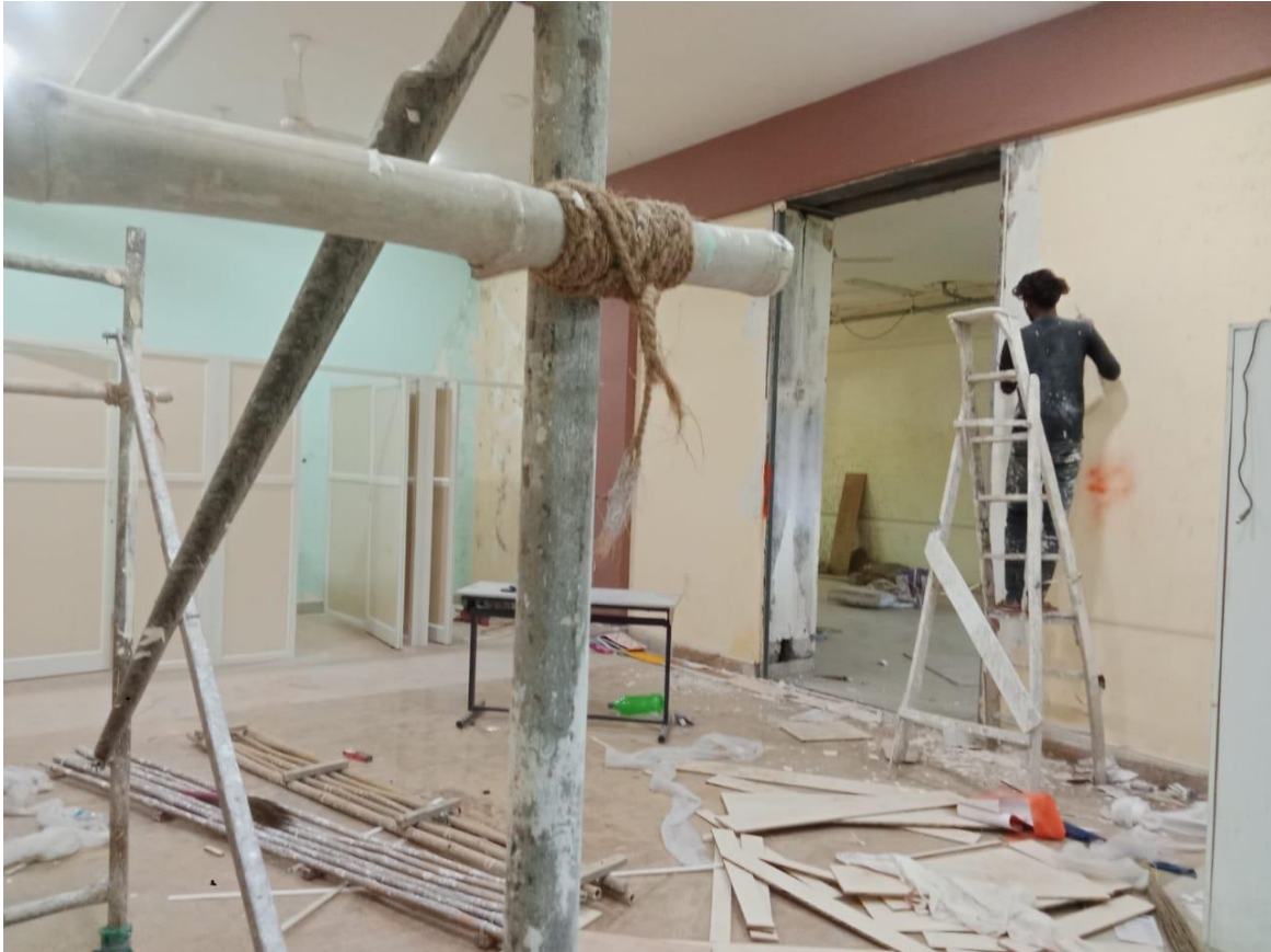
Painting work at first floor of college building
